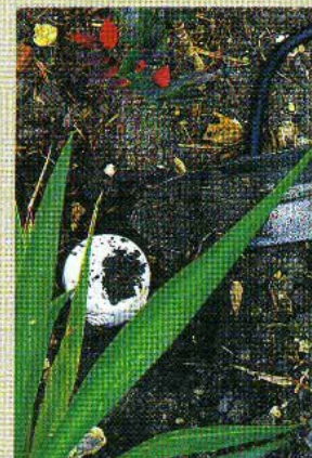
ABOVE: Burying junction box
