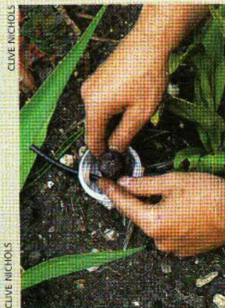
ABOVE: Putting sealant into the junction box
